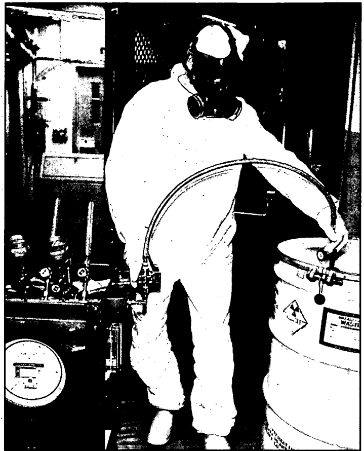
A Rocky Flats worker vents a mixed waste drum, to relieve any buildup of potentially-explosive hydrogen gas.
