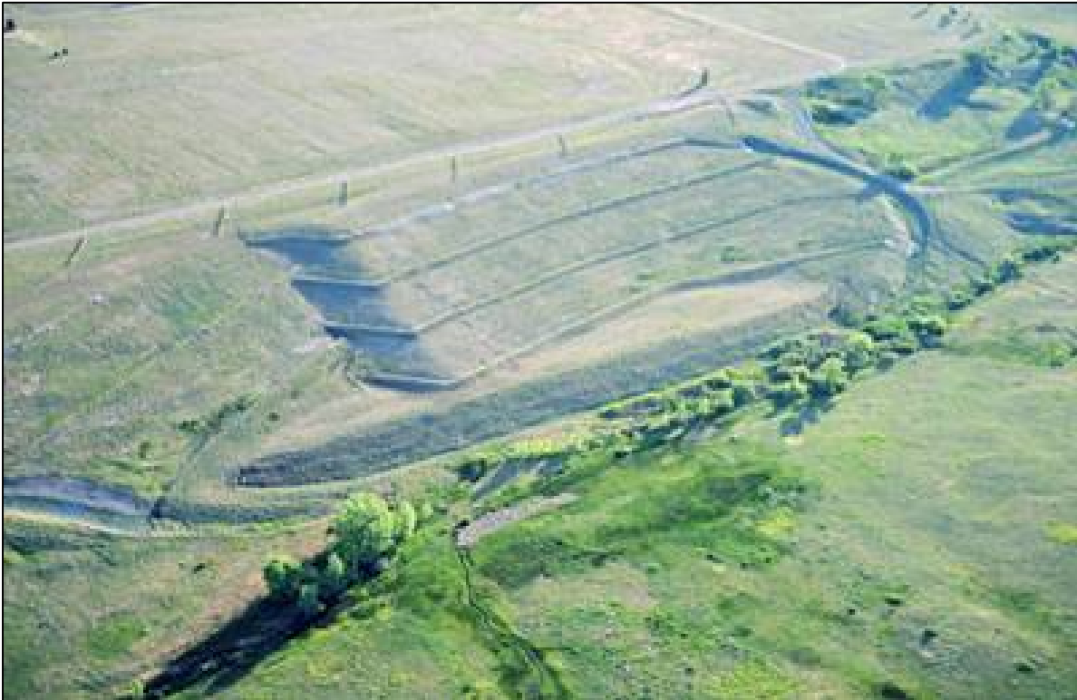
Photograph D9. Aerial photograph of the Original Landfill
