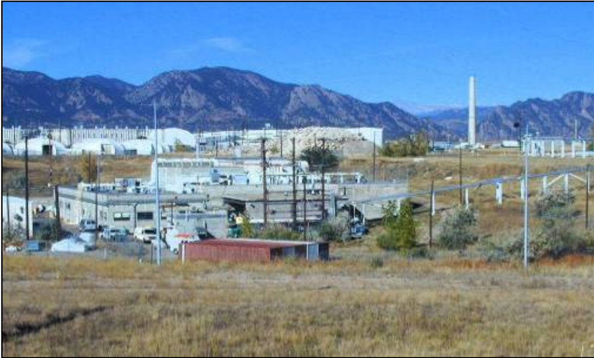
Photograph D5. B991, 700 Area in background, 2003
