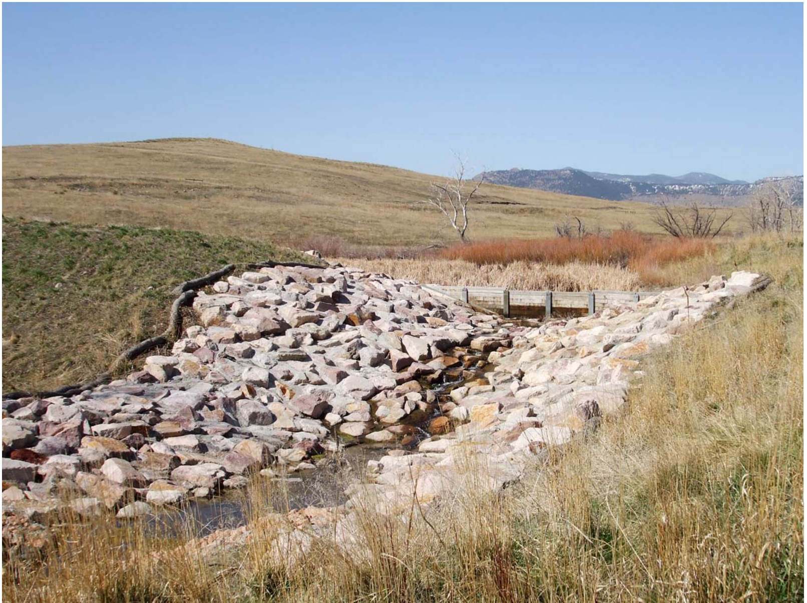
Figure 4. Example of Notched Dam with Stoplog Structure and Grouted Riprap
