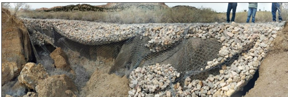
Figure 7: Damage from Erosion at the DOE Office of Legacy Management’s L-Bar Site in New Mexico
