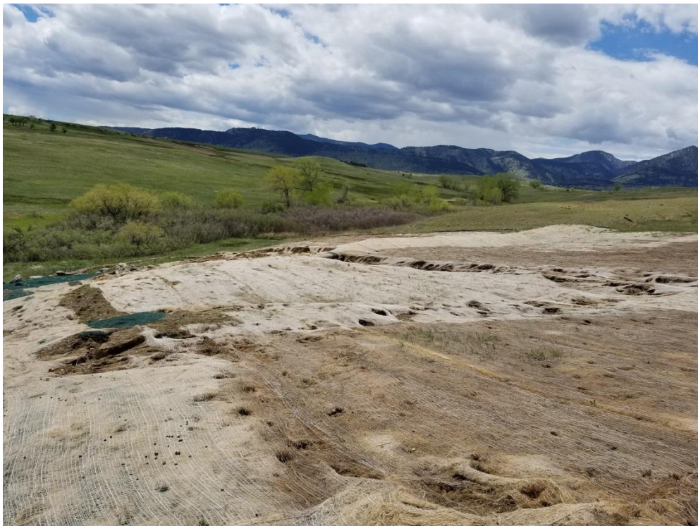
Figure 2: Looking Southwest Towards the Recent Slump from the Berm 6 Outfall
