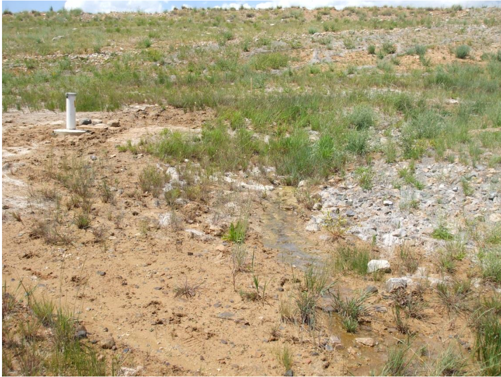
Figure 9: Looking Northwest at the Small Gully Discovered Below Seep 10
