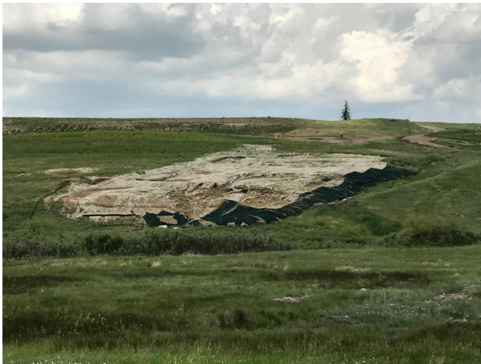
Figure 2: Looking North Toward Slump, Taken 6/13/2017.
