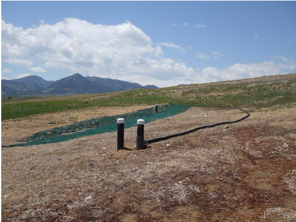
Figure 7: Looking West at Berm 4 and the Gravity Drain Line Connection to the ESSD Pictured as the Black Risers
