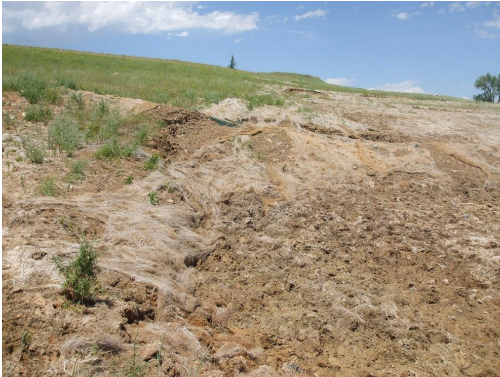
Figure 3: Looking North at the New Crack That Runs Through Berms 6 and 7
