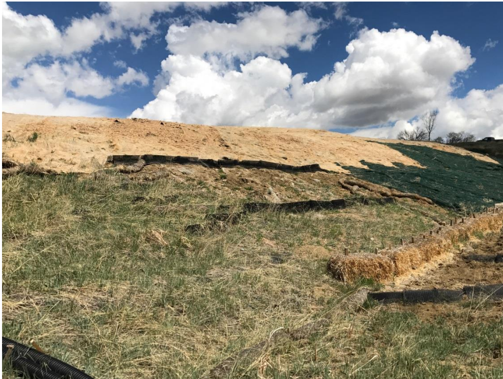
Figure 5: Standing on the EPC Outfall Looking North at Berm 7
