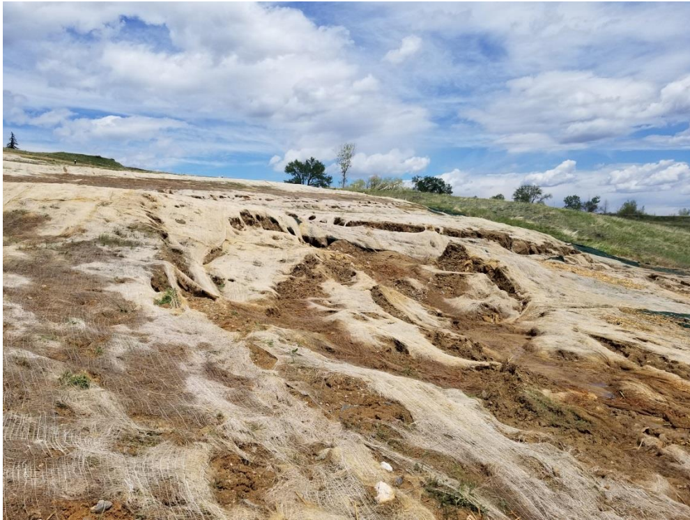
Figure 4: Standing at the EPC Outfall Looking North at Berm 7
