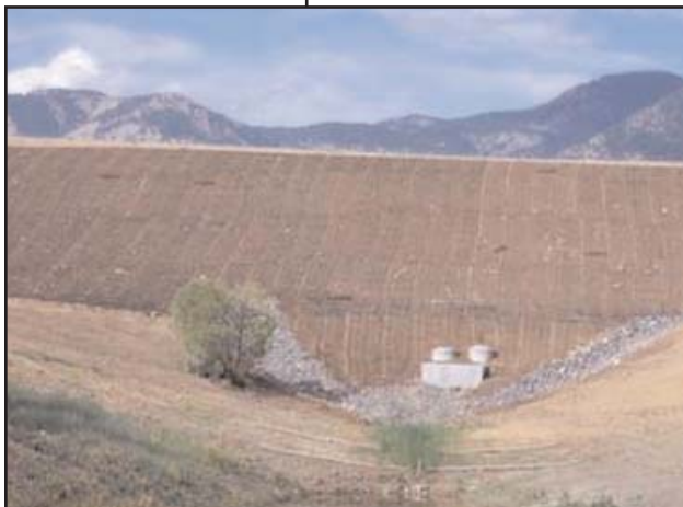
A large earthen cap was constructed over the Present Landfill at Rocky Flats.
